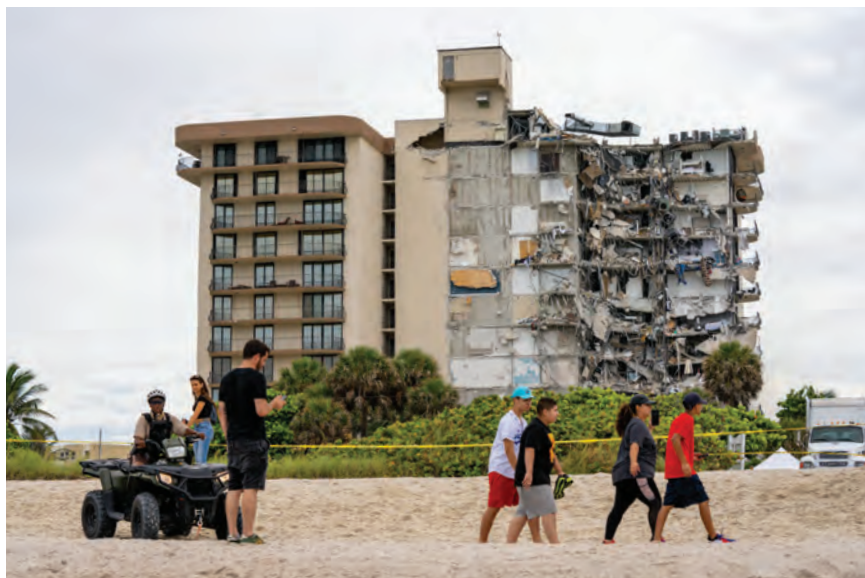
Part of the 12-story oceanfront Champlain Towers South condominium, which collapsed around 2 a.m. on Thursday, June 24, 2021.
